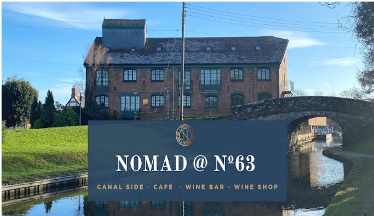
- View of premises from canal, South West (Nomad @ 63 internet photo) -
