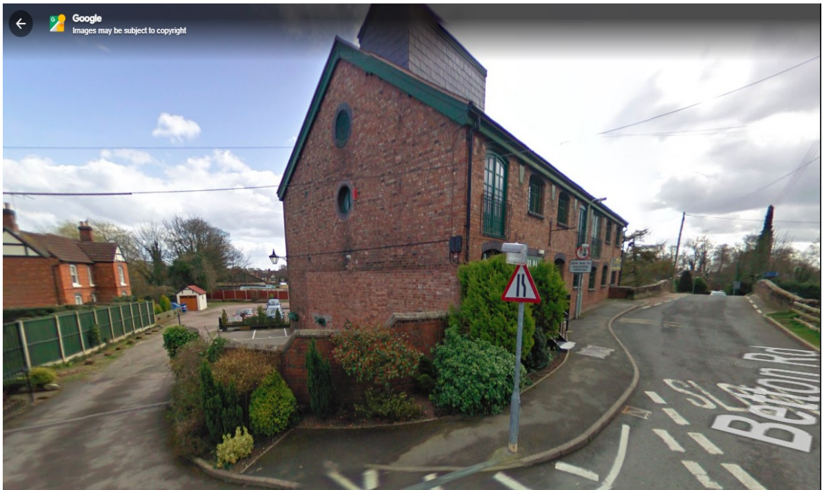
- Side view of premises, Betton Road and Waterside Drive junction -
